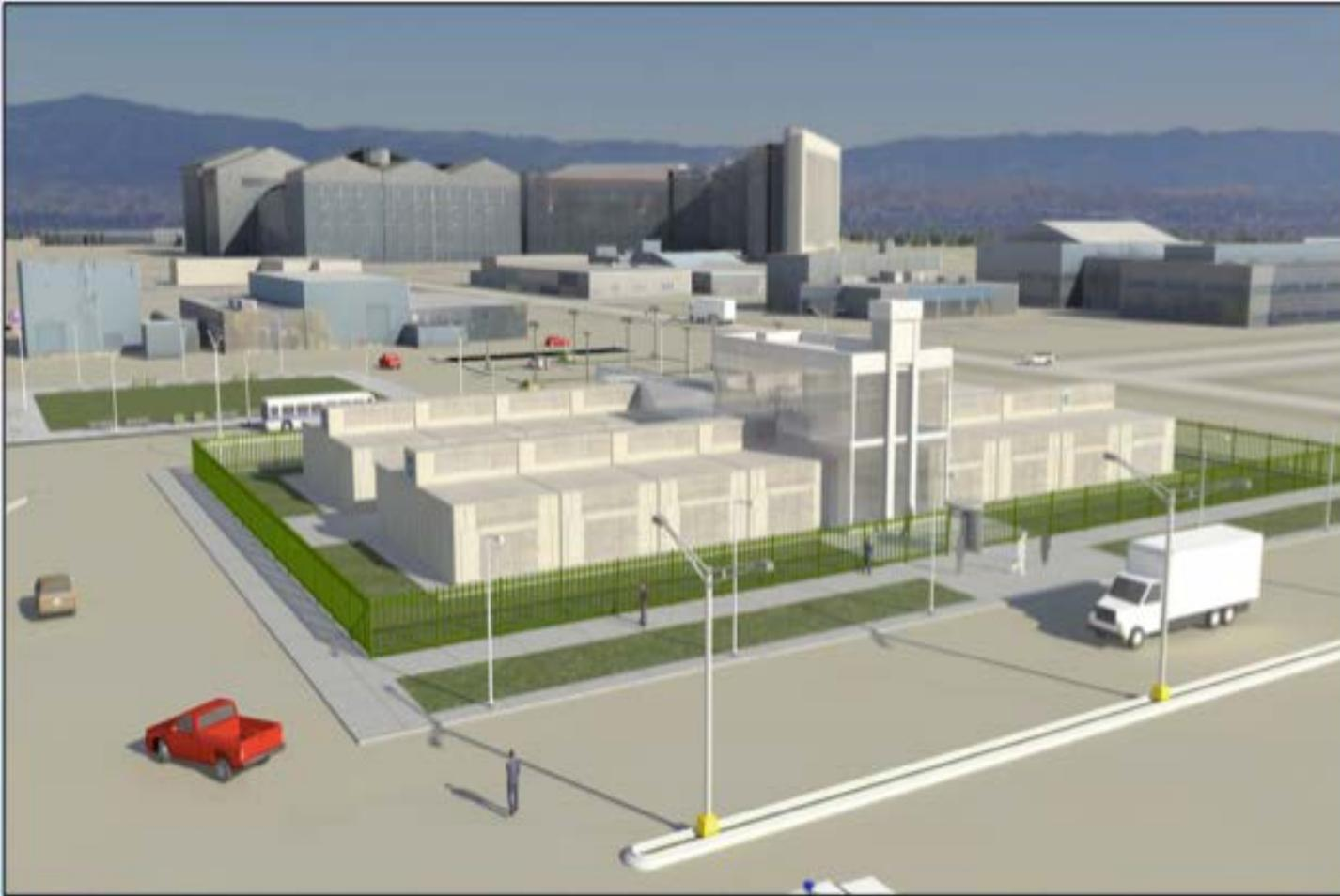
This artist rendition shows a possible full deployment of a Modular Supercomputing Facility. Capable of housing 256 compute racks or 18,432 nodes this would have almost 100 more racks than Pleiades and use just over 6MW of power. The cost estimate which is being refined would be under \$40M for the site preparation and all of the modules.
